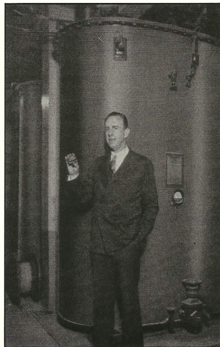
Here Powel Crosley, Jr. is holding in his hand one of the smallest audio transformers formerly in use for WLW. Behind him is seen a portion of the huge audio transformer used in connection with the 500,000 watt transmitter. It weighs over 35 tons and is, by far, the largest in the world.
